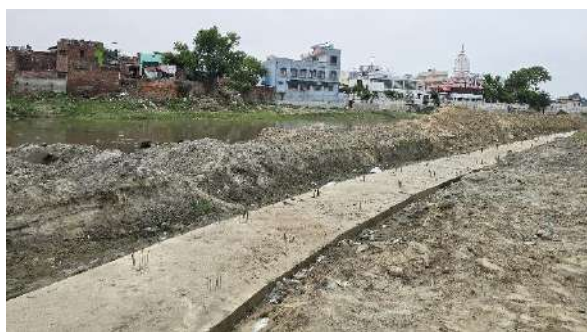
Image 6-17: Ongoing construction of retaining wall for pathway
