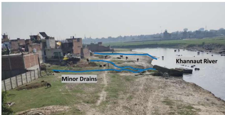
Image 6-2: Sewage outflow along with minor drain after intercepting the Lodhipur drain
