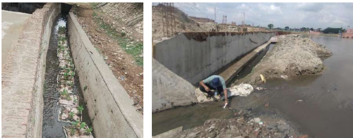
Image 4-2: Phyto-remediation at Ahmedpura Reti drain
